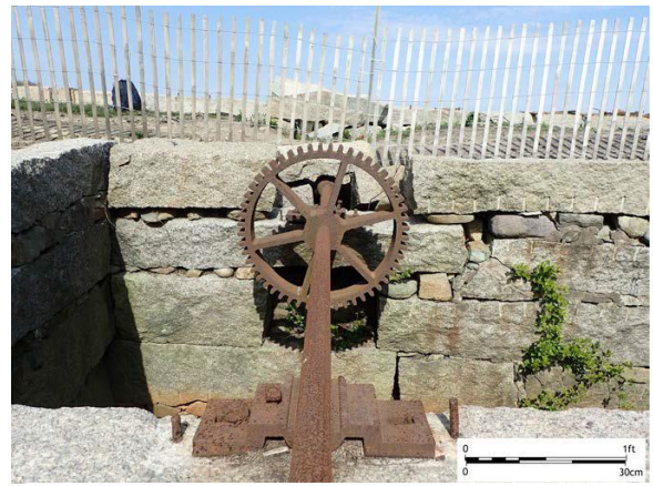
Figure 10: Pinion gear, shaft and bearing to power line shaft in Lower Yard (PAL photo)
