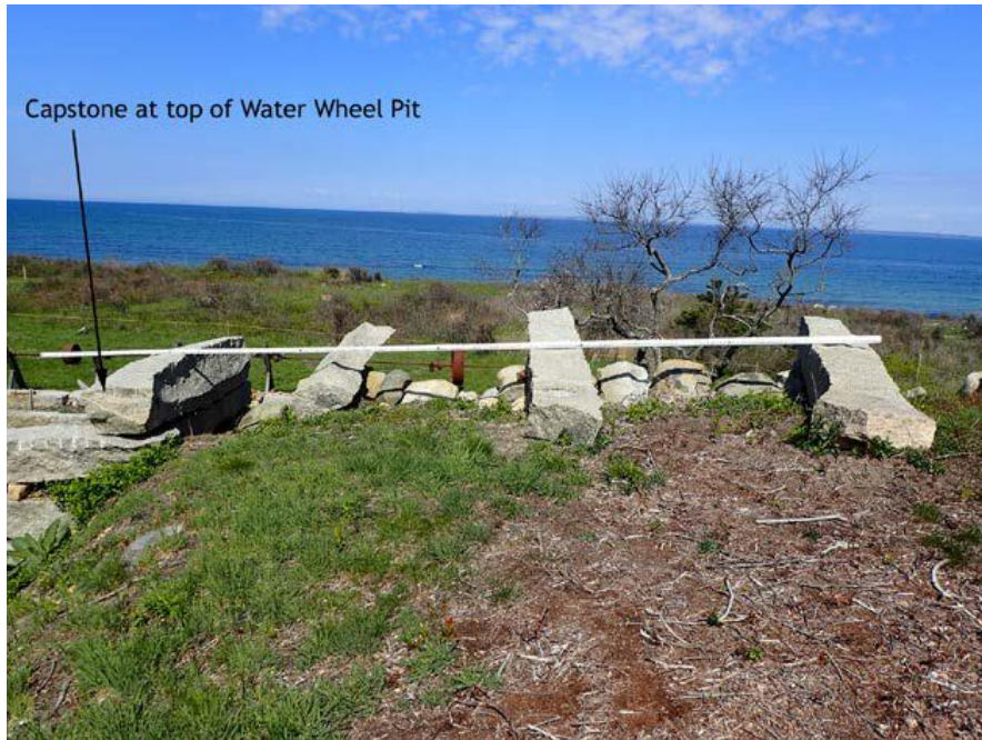
Figure 13: Cantilevered granite blocks indicating former support of flume (PAL photo)
