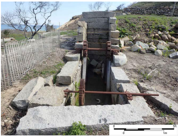
Figure 12: Water wheel pit and gears (PAL photo)
