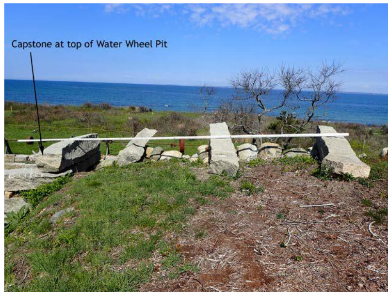
Figure 9: Cantilevered granite blocks indicating former support of flume (PAL photo)
