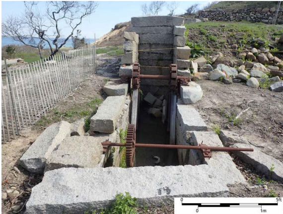
FIGURE 8: WATER WHEEL PIT AND GEARS (PAL PHOTO)
