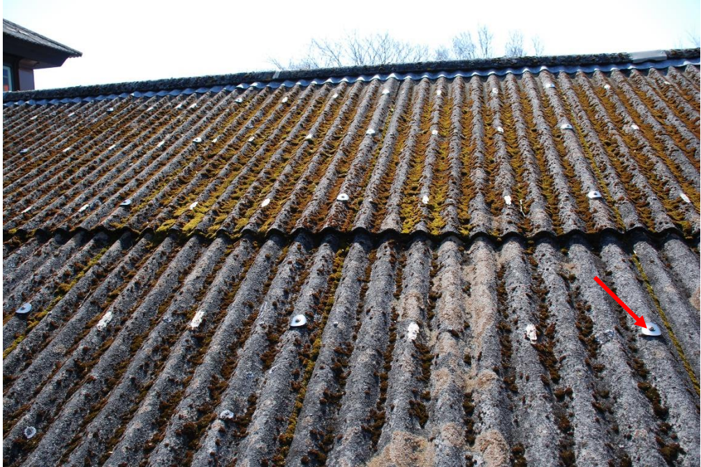
Photo 4 - View of Cement-Asbestos sheet roofing. Note: face fasteners.
