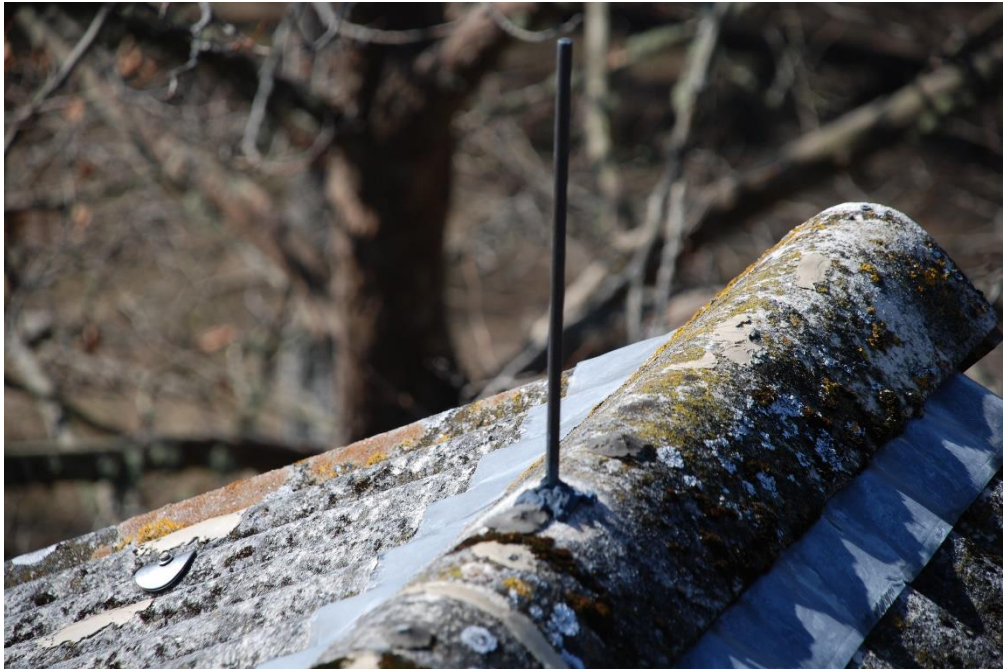
Photo 28 - View of old lightning protection aerial.
