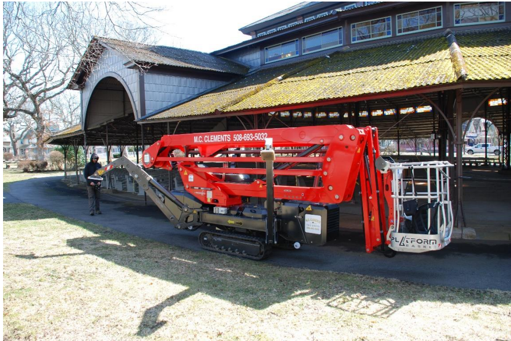
Photo 1 - View of articulating boom lift provided by M.C. Clements Tree Service.
