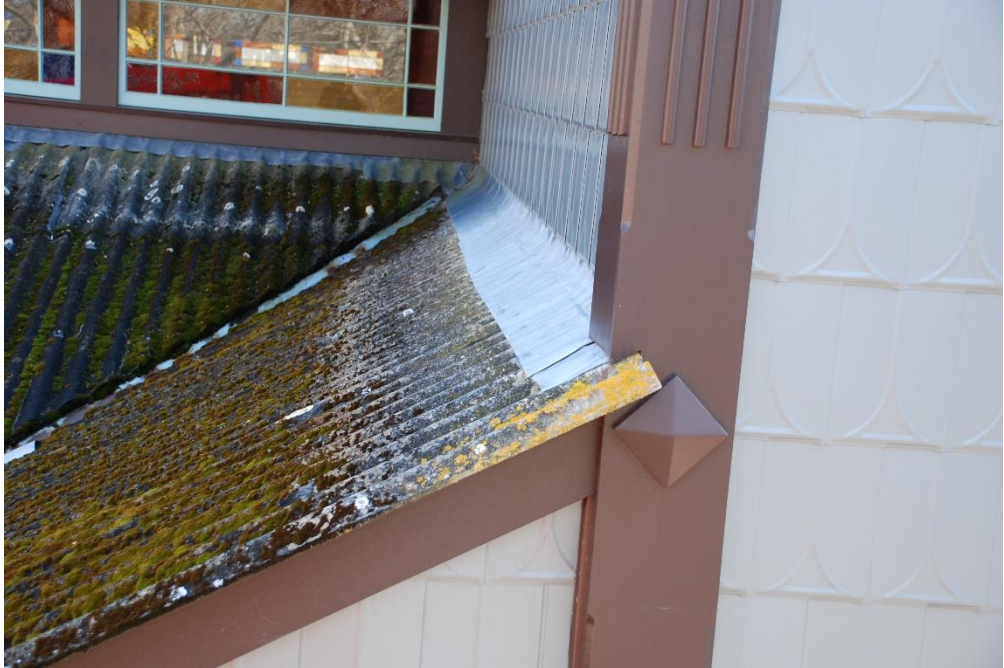
Photo 24 - View of base flashing at vertical wall to roof interface.
