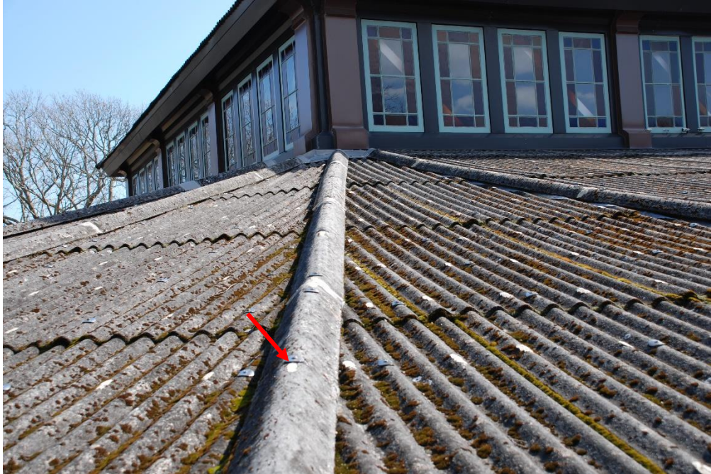
Photo 13 - View of typical roof hip cover. Note face fastener.
