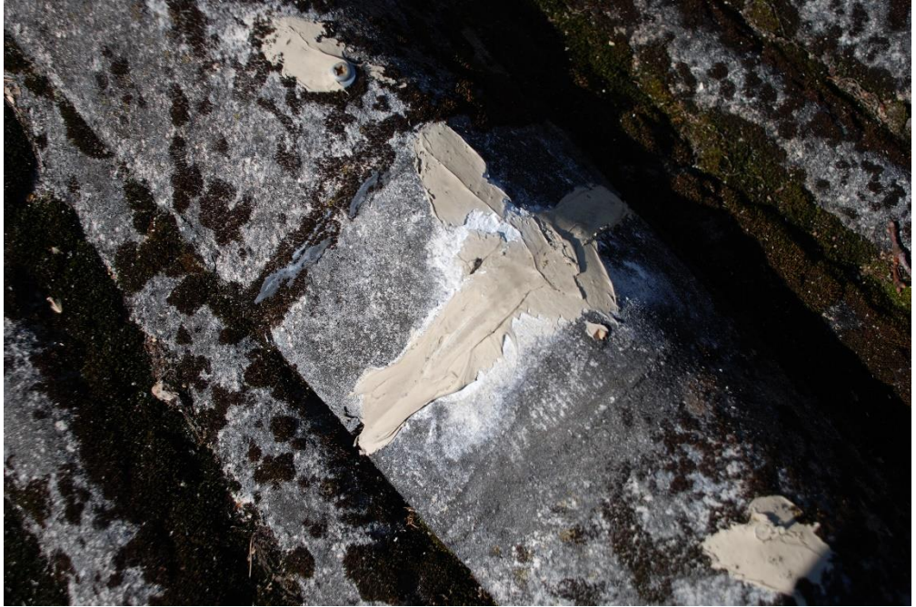
Photo 21 - View of sealed crack in hip cover.
