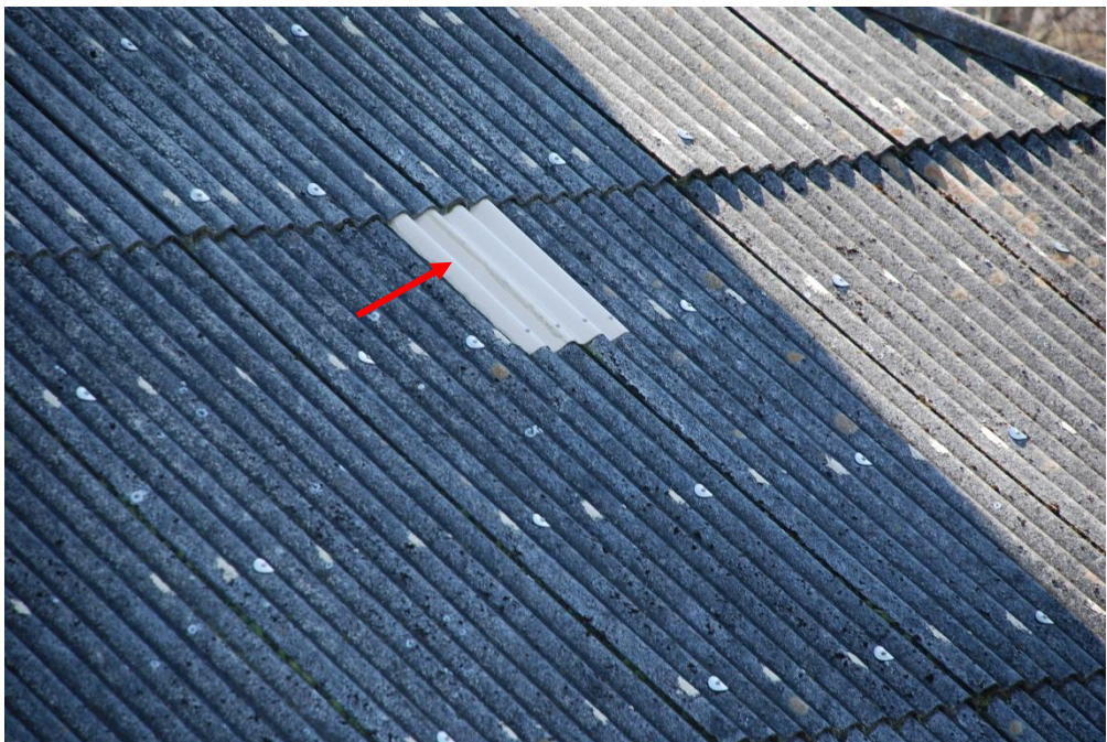
Photo 12 - View of patch covering hole in cement-asbestos panel (exterior side).
