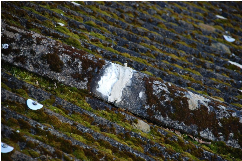
Photo 20 - View of sealed crack in hip cover.
