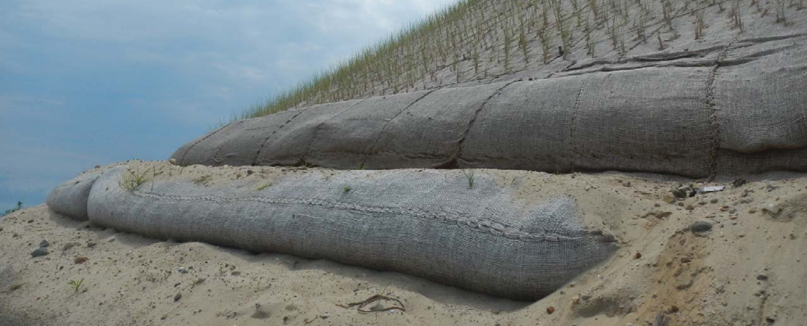
Sconset Bluff Protection Coastal Engineering and Modeling
