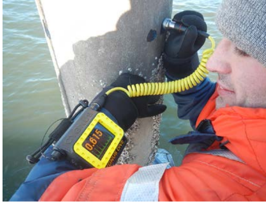
Photograph #1: UTM Reading on steel pile
