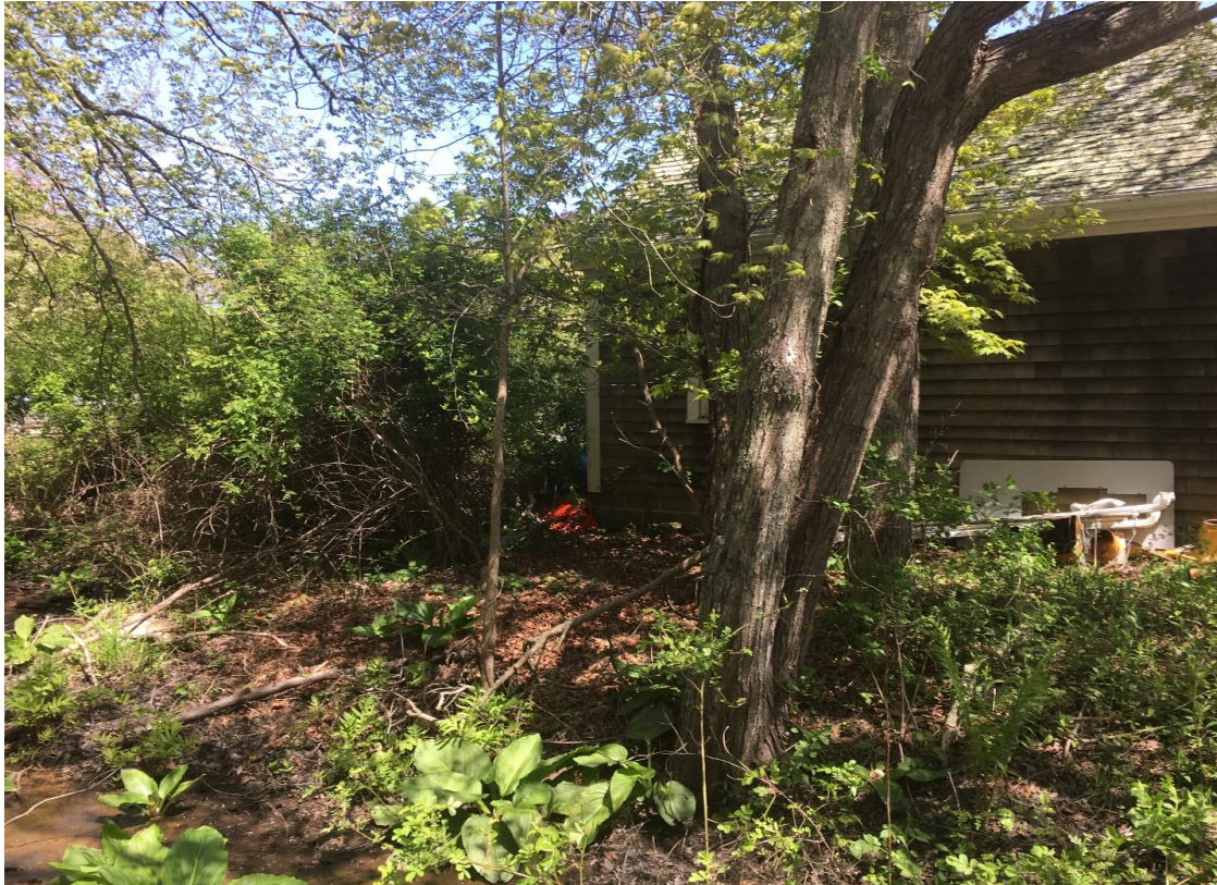
Photo 5: EMS building located adjacent to wetlands.
