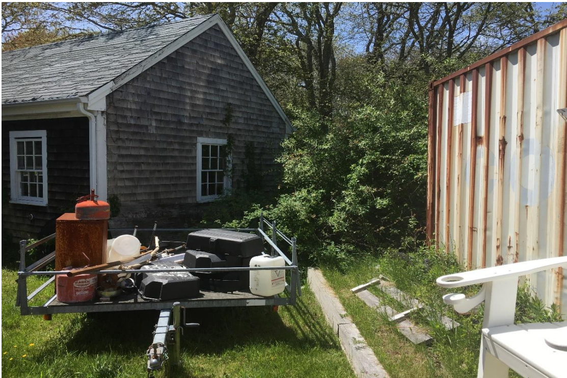
Photo 4: Storage container and rear of EMS building adjacent to wetlands.
