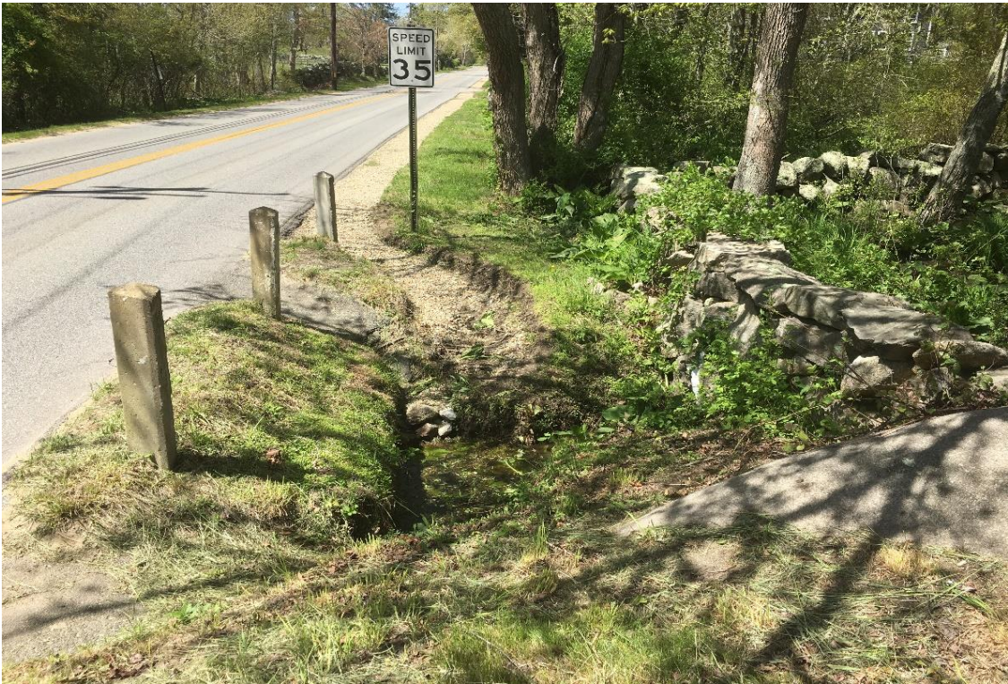
Photo 2: Intermittent stream at mouth of culvert beneath Menemsha Crossroad.
