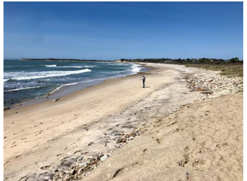
Figure 8. Fool's High Tide cobble berm construction complete, May 2020
