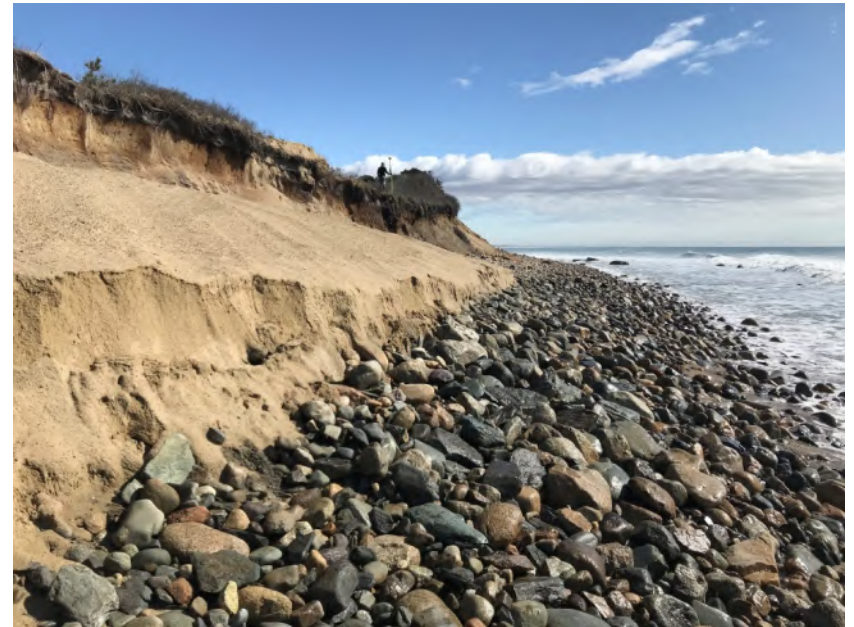
Figure 4. FHT cobble berm reconstruction complete, April 1, 2022
