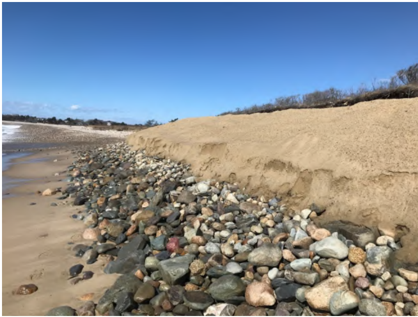
Figure 9. FHT cobble berm reconstruction complete, April 1, 2022
