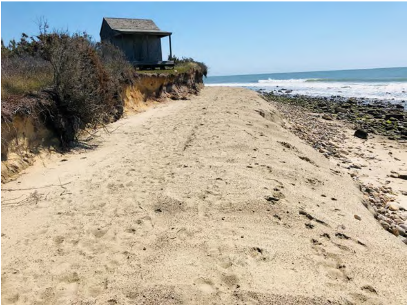
Figure 7. Fool's High Tide cobble berm construction complete, May 2020
