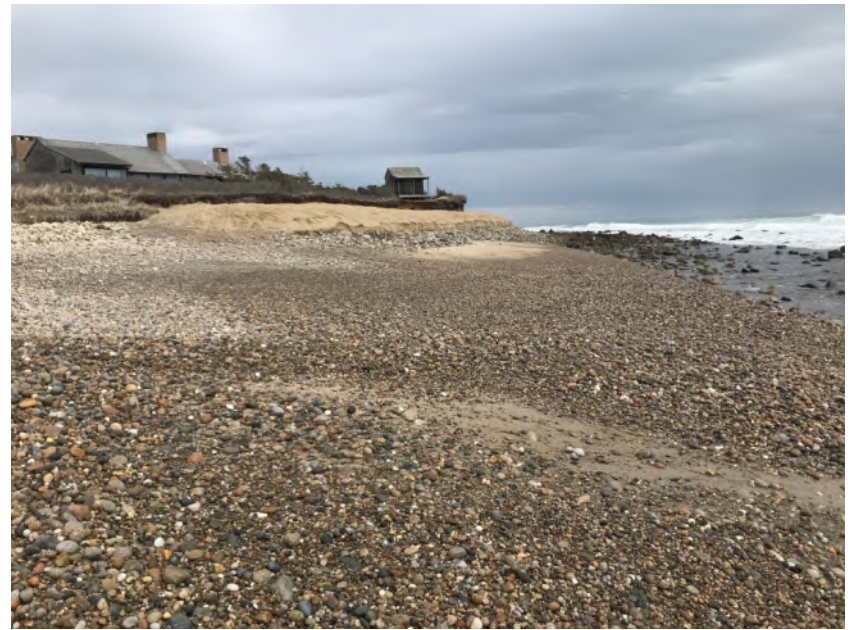
Figure 2. FHT cobble berm reconstruction complete, April 1, 2022
