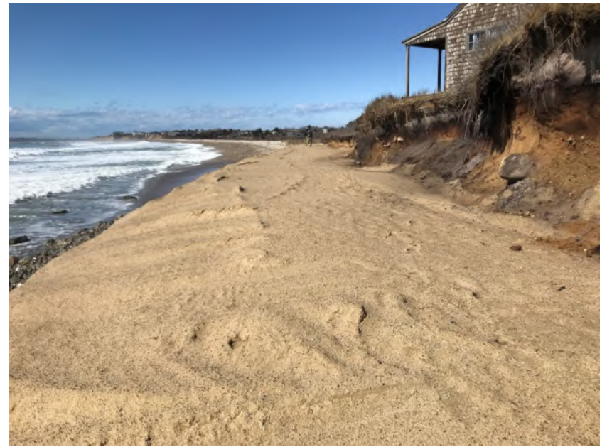
Figure 6. FHT cobble berm reconstruction complete, April 1, 2022
