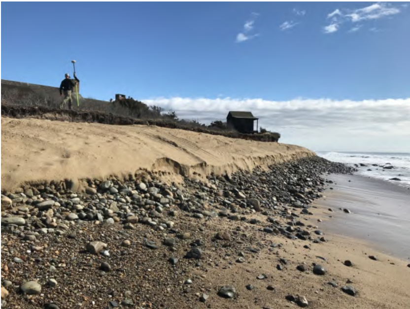
Figure 3. FHT cobble berm reconstruction complete, April 1, 2022
