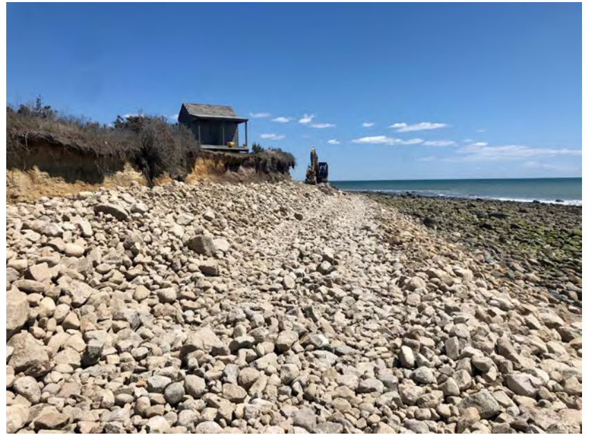
Figure 6. Fool's High Tide cobble berm construction, May 2020
