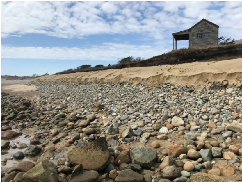
Figure 7. FHT cobble berm reconstruction complete, April 1, 2022
