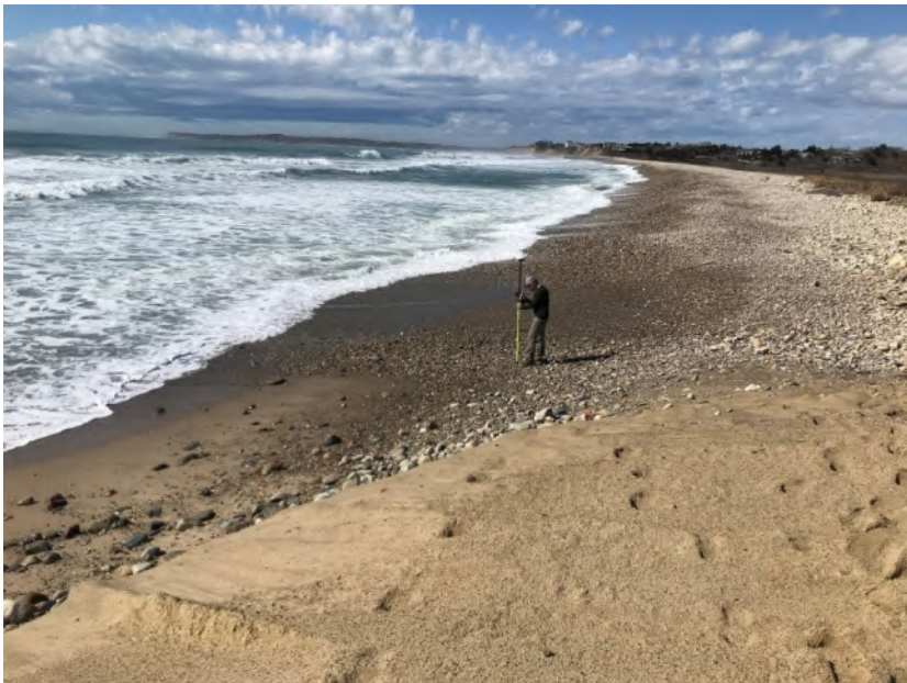
Figure 11. FHT cobble berm reconstruction complete, April 1, 2022
