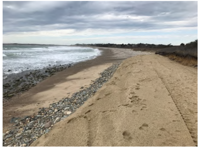
Figure 10. FHT cobble berm reconstruction complete, April 1, 2022
