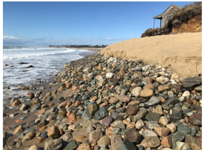
Figure 8. FHT cobble berm reconstruction complete, April 1, 2022
