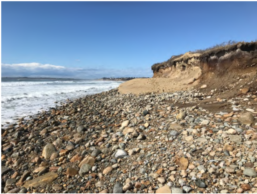
Figure 5. FHT cobble berm reconstruction complete, April 1, 2022
