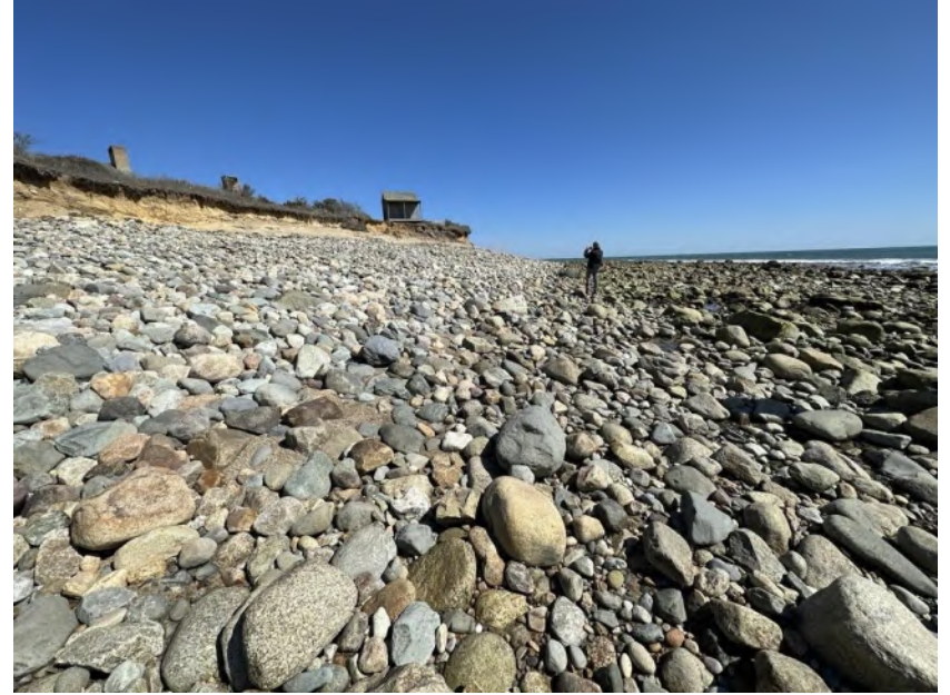
Figure 5. FHT beach and exposed coastal bank, March 20, 2023
