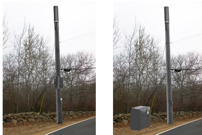
The above images show how the equipment will appear—and the minimal impact it will have on Island aesthetics.
