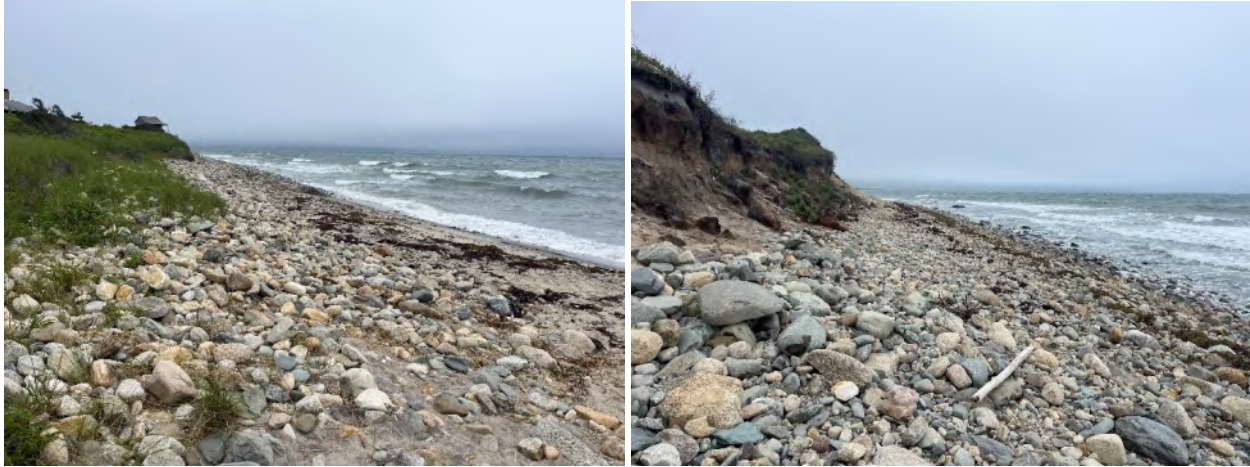
Figure 2. July 10, 2023 photos showing site conditions. Left – Photo from the southwest property boundary looking northeast along 25 East Lane. Right – Photo from farther along the beach, looking northeast along 25 East Lane towards 21 East Lane.
