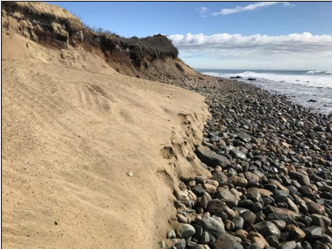
Figure 5. Photo looking east at the eastern taper of the constructed cobble berm – April 1, 2022. The subject property and footprint of the proposed project is an extension of the constructed design along the unprotected bank in the distance of this photo.
