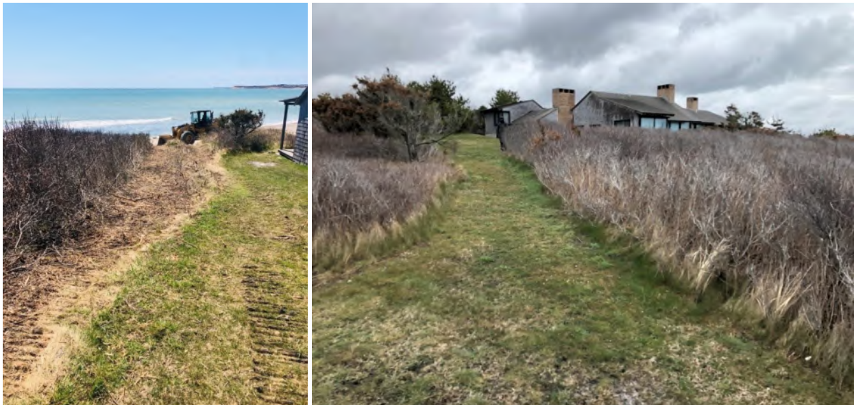
Figure 14. Photographs showing construction access way through 25 East Lane for construction equipment – May 2020.
