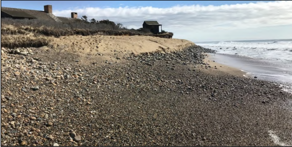
Figure 4. Photo looking east along the second constructed cobble berm at 25 East Lane – April 1, 2022.
