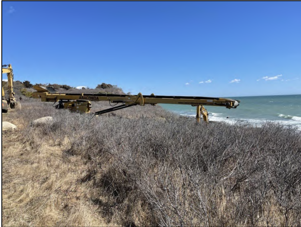
Figure 50. Photograph showing the use of a conveyor belt to transport material over the bank at 21 East Lane.
