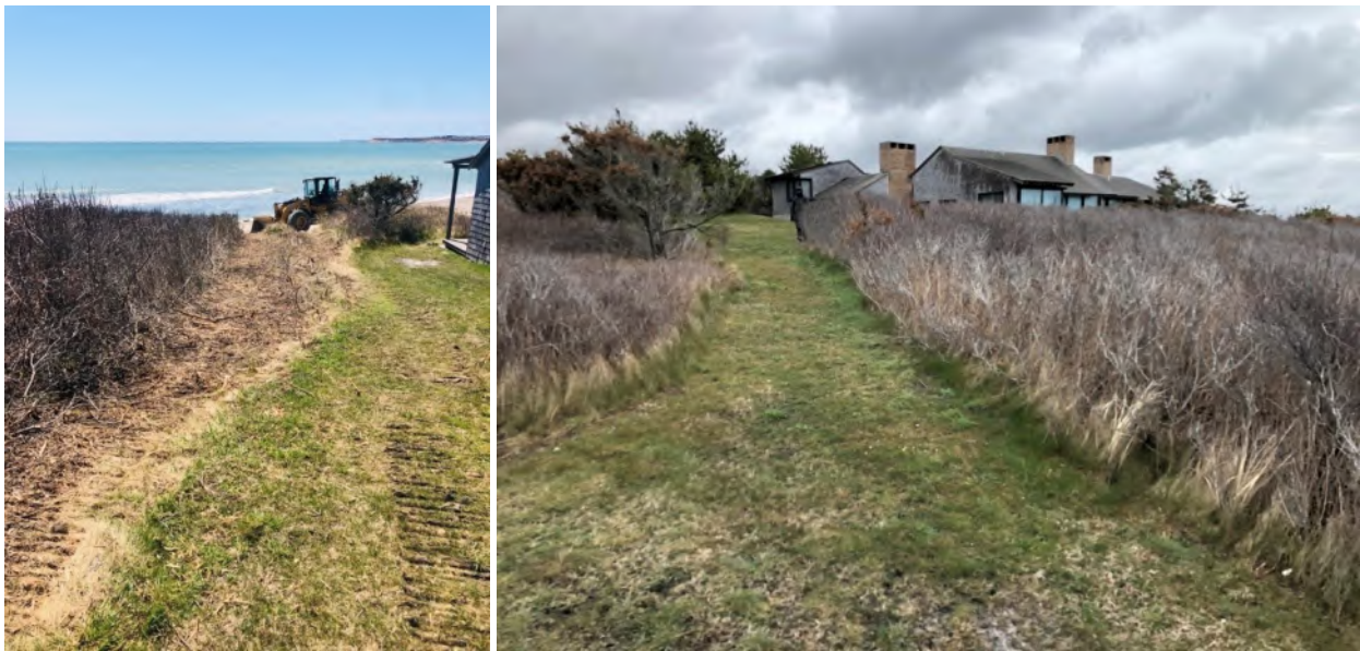
Figure 72. Photographs showing construction access way through 25 East Lane for construction equipment – May 2020.
