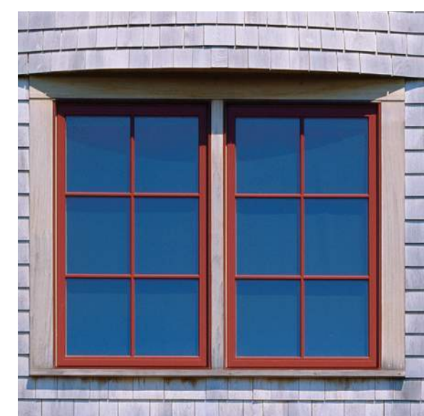
PRE-FINISHED ALUMINUM CLAD WINDOWS
