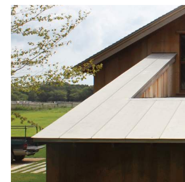
ZINC COATED COPPER STANDING SEAM ROOF
