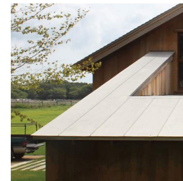
ZINC COATED COPPER STANDING SEAM ROOF
