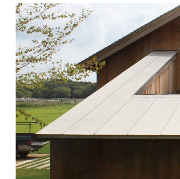
ZINC COATED COPPER STANDING SEAM ROOF
