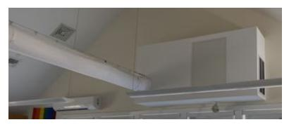
units use a set of fans to bring fresh air from outside and exhaust from inside simultaneously. An internal heat exchanger allows the energy from inside the building to be transferred to the air from the outside, which reduces the demand on the heating system. These units were installed in custom fabricated boxes and mounted either high on the wall in high ceiling areas or on the ceiling in flat ceiling areas. The supply air is distributed to the space with a fabric duct.
