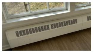
Overall, the heating system is inadequate; largely because it was never intended as the sole source of heat. The original design intent was for the finned tube radiation and the air handling units to jointly provide the heating and ventilation for the spaces. Once the air handling units were disconnected, the sole source of heat remaining was an undersized finned tube radiation system. In addition to being undersized, the layout of the radiators does not allow for complete heating coverage
