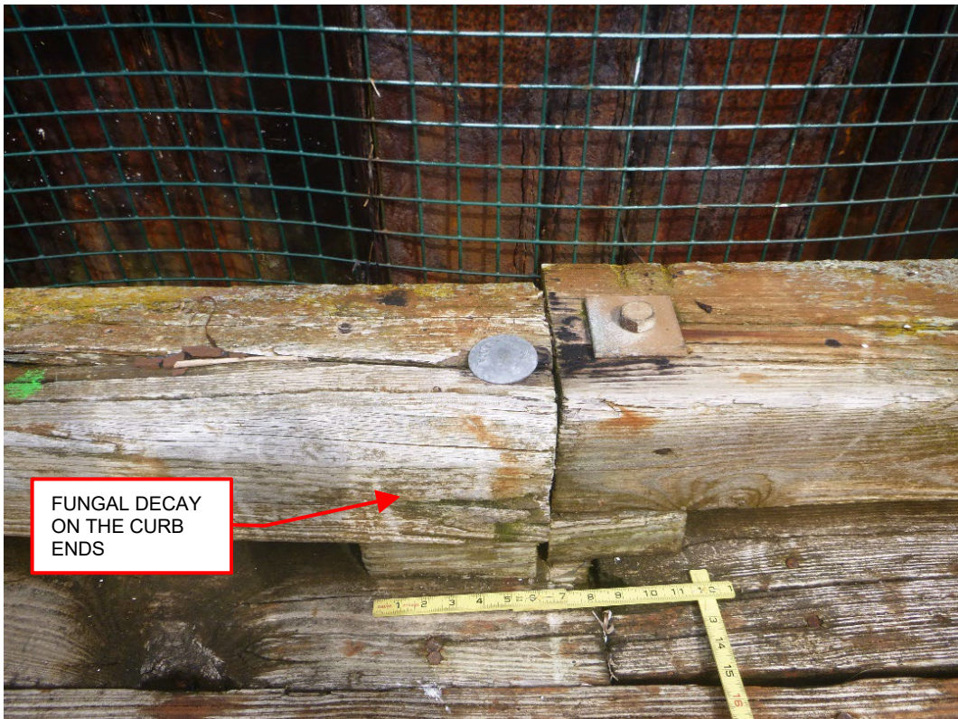
Photo 32 – Close up of the fungal decay on the curb.
