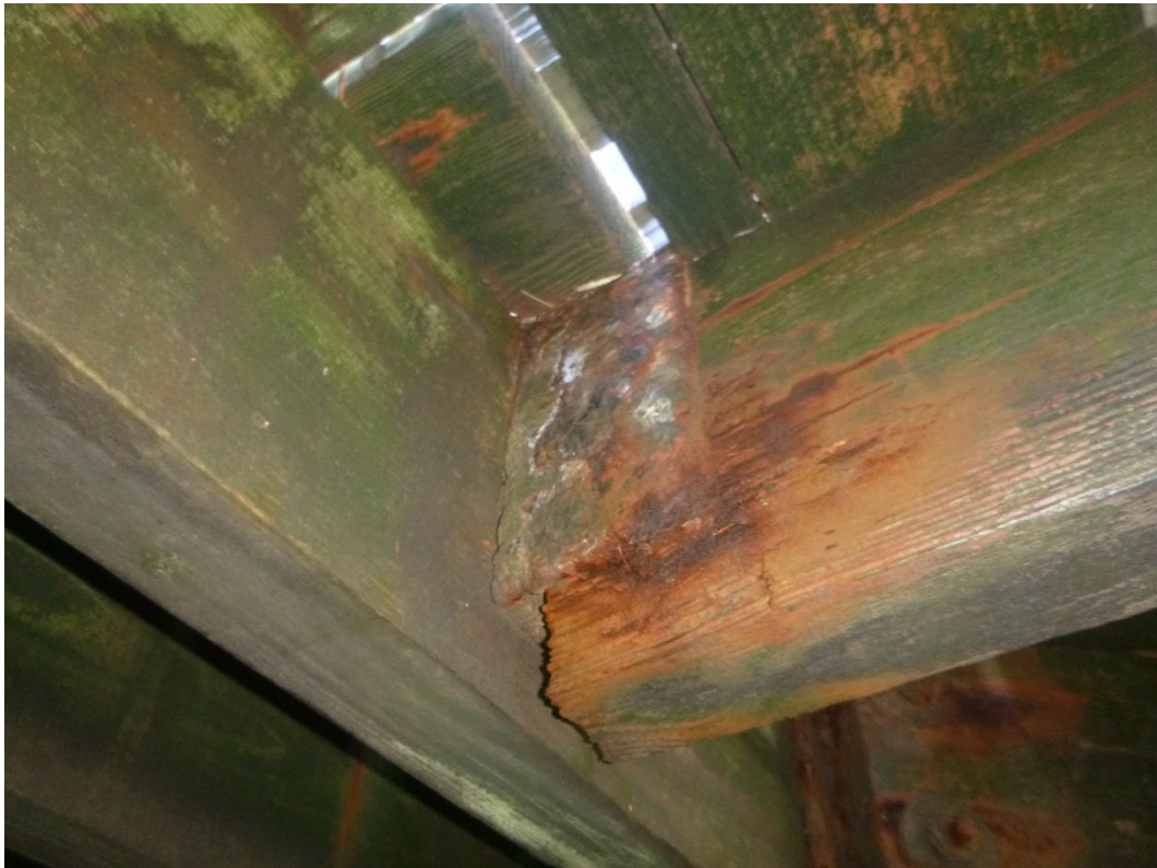
Photo 23 – Close up of the butt connection between Bents 6 and 9.
