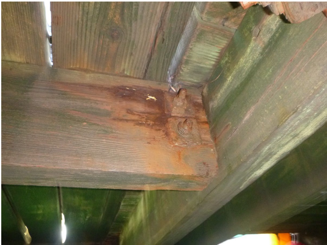
Photo 24 – Close up of the butt connection between Bents 6 and 9.
