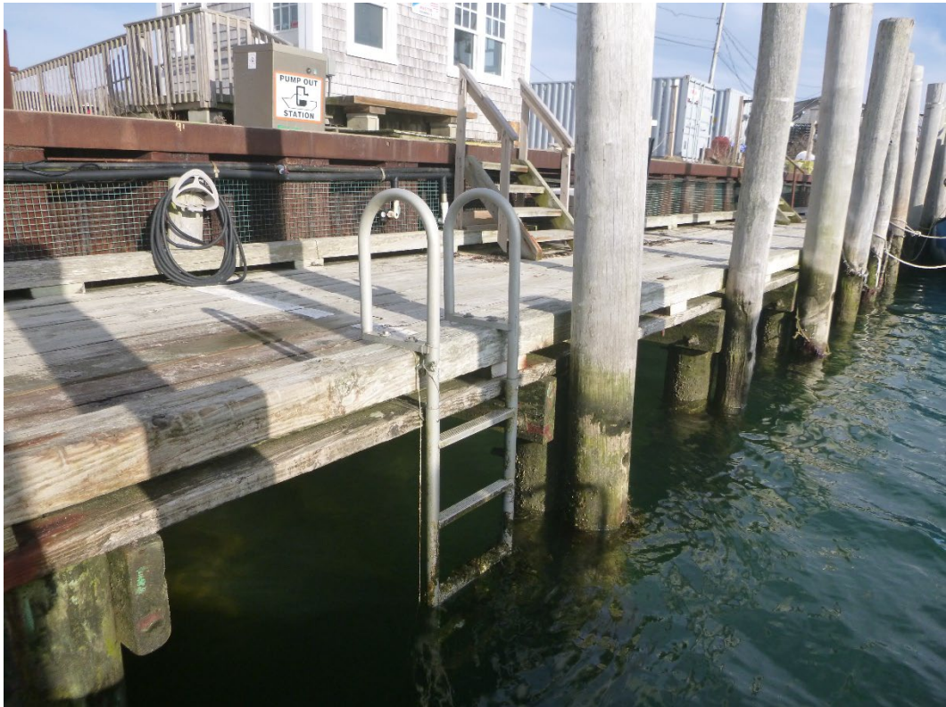
Photo 2 – General view of the wharf construction.
