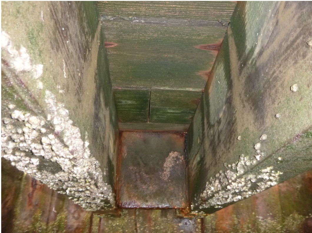
Photo 26 – Typical view of the steel channel connecting to the sheet pile.
