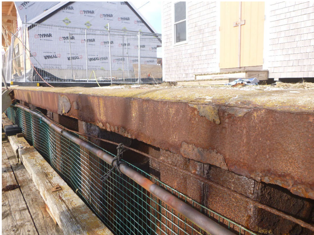
Photo 12 – Typical view of the steel sheet pile cap.
