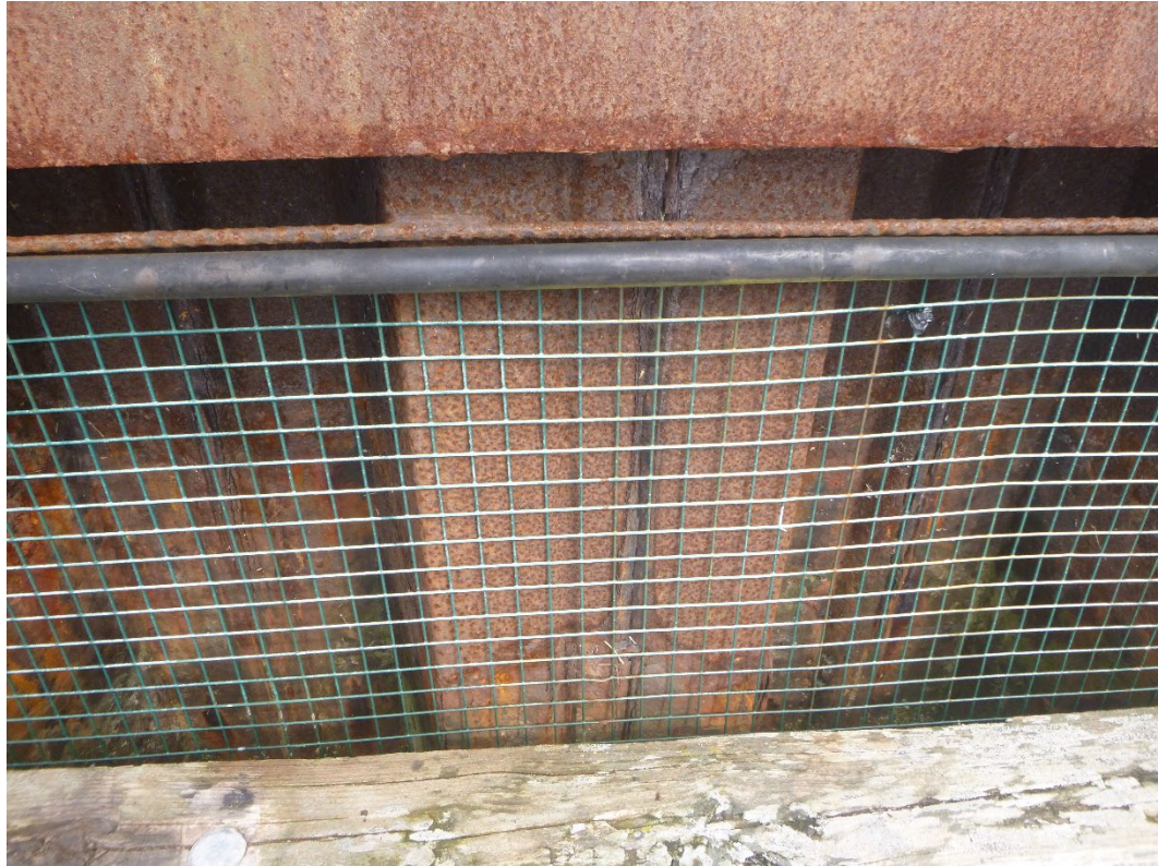
Photo 3 – Typical view of the steel sheet pile bulkhead.
