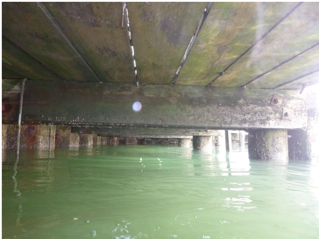
Photo 18 – Underdeck view of the timber split cap.
