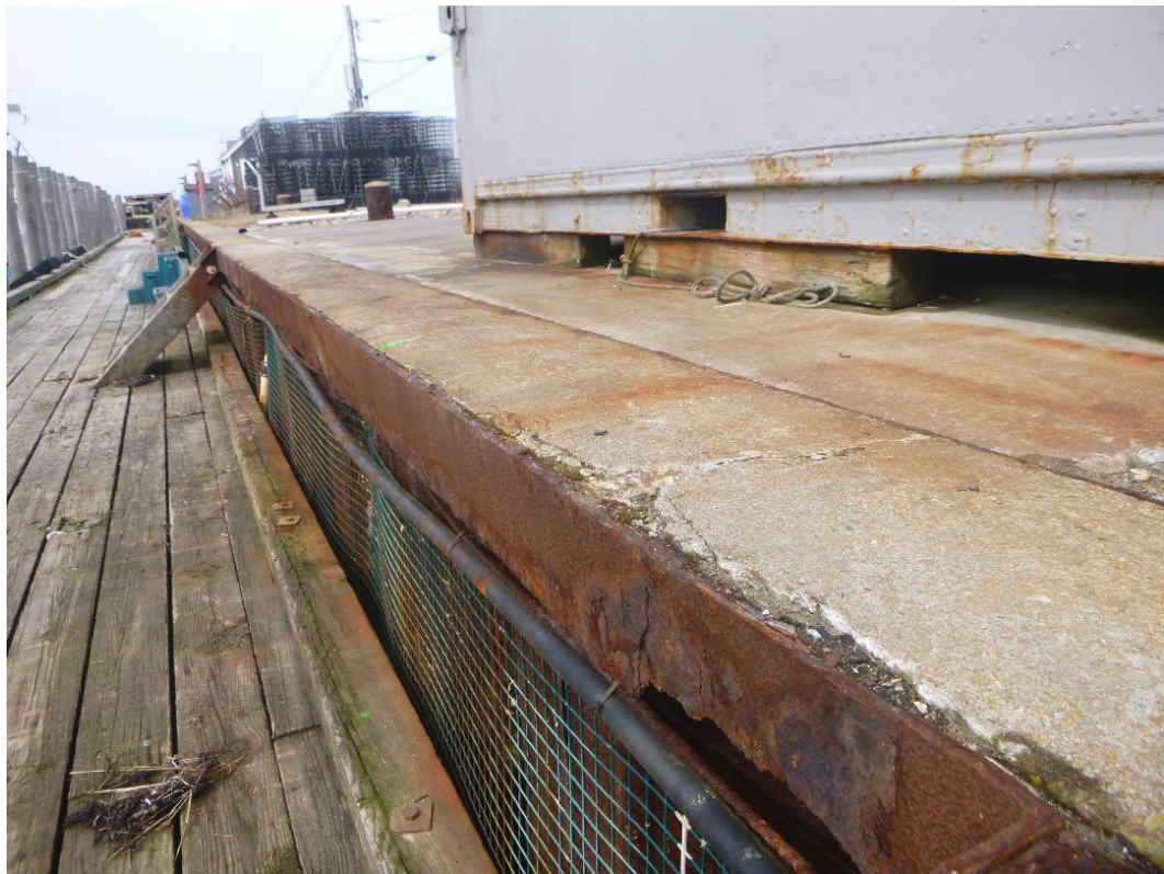
Photo 14 – The concrete with minor deterioration.
