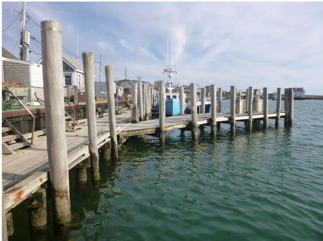
Photo 36 – Overall view of the Fuel Pier.
