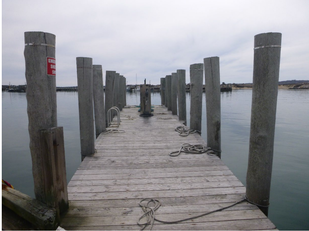
Photo 37 – Overall view of the Fuel Pier.
