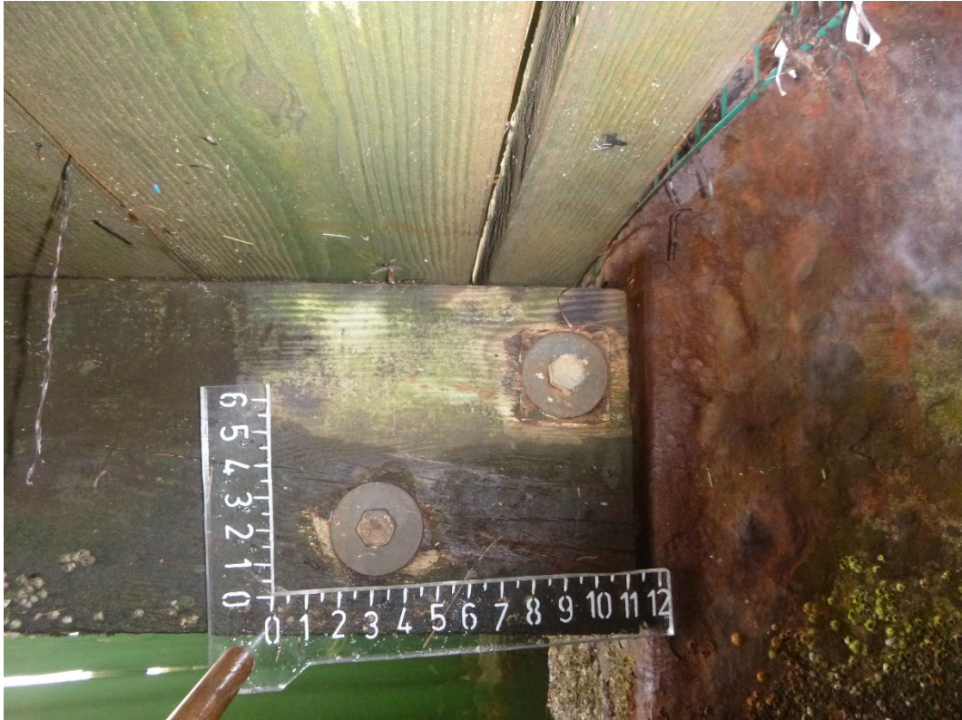
Photo 27 – Through-bolts connecting the pile cap to the channel.
