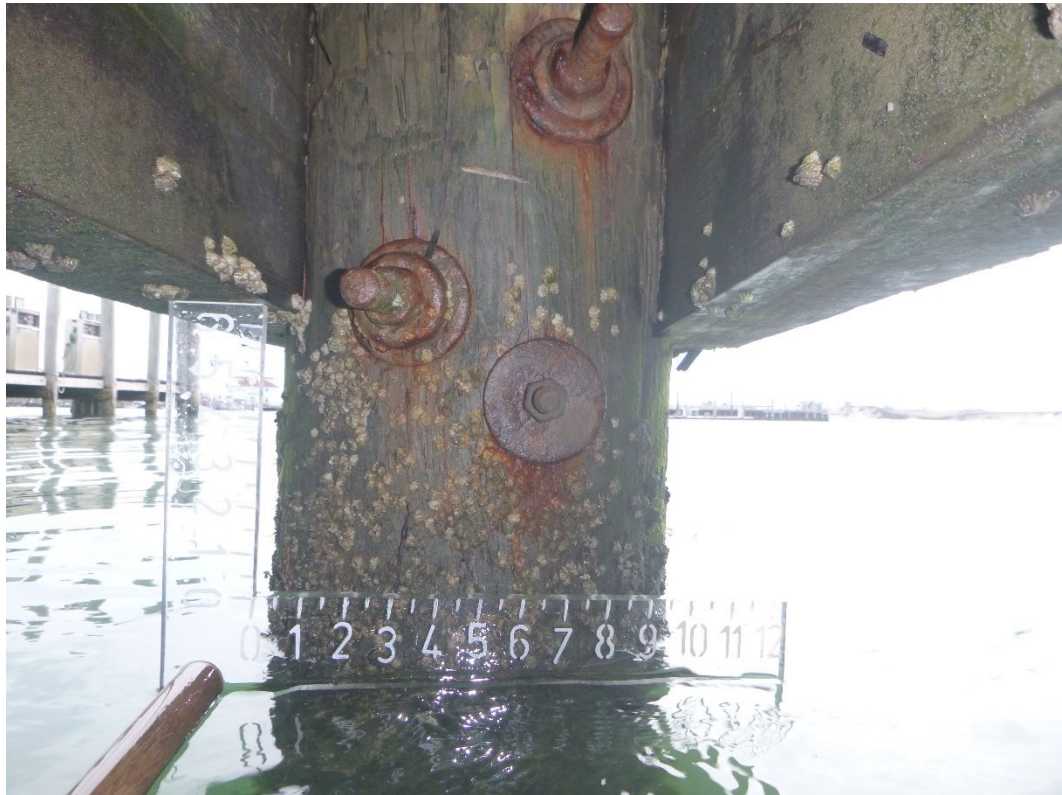
Photo 16 – Timber fender pile connection to the piles supporting the wharf.
