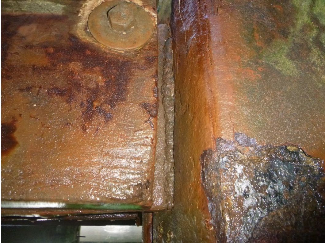
Photo 29 – Close up of the steel channel to sheet pile weld.
