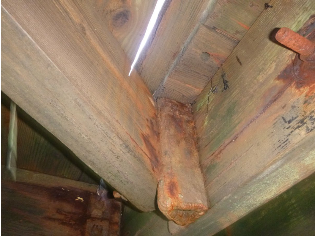
Photo 25 – Underdeck view of the timber split cap.
