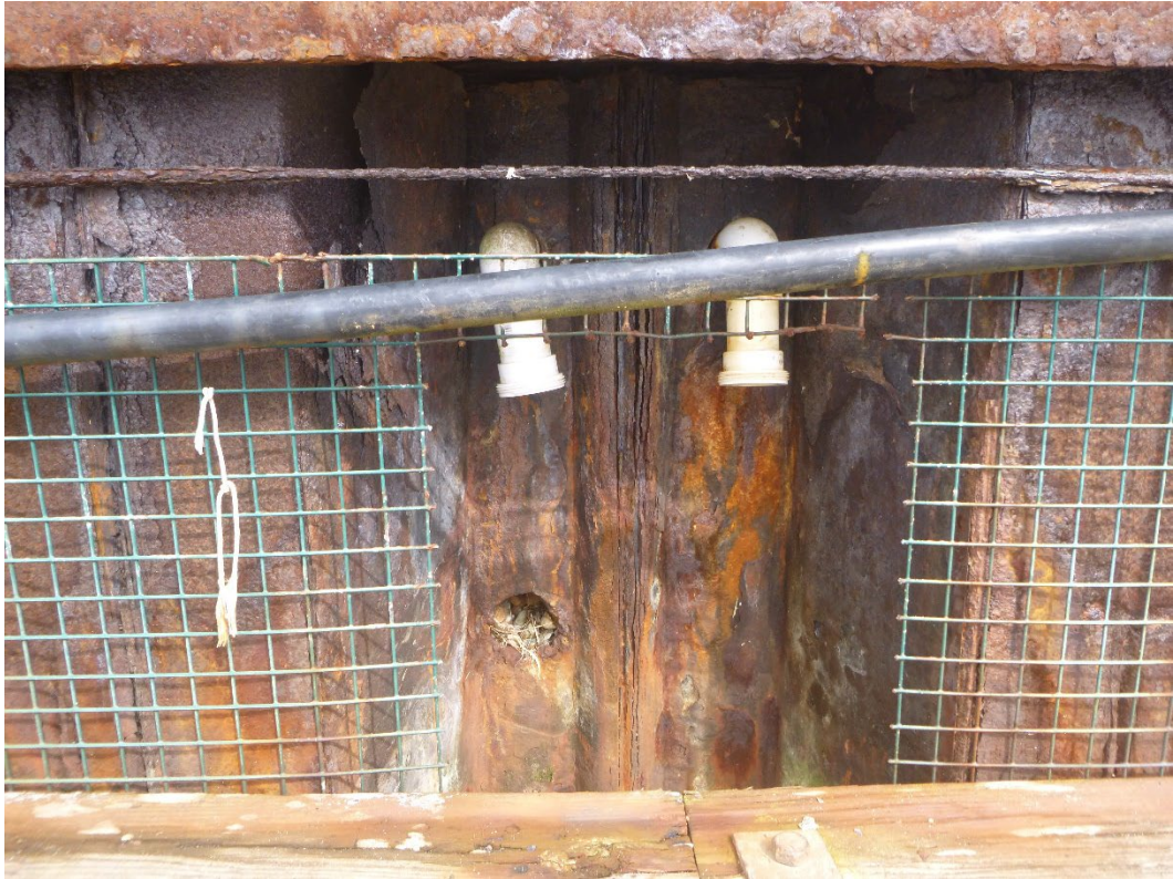
Photo 39 – Intake and outfall pipes through the sheet pile.
