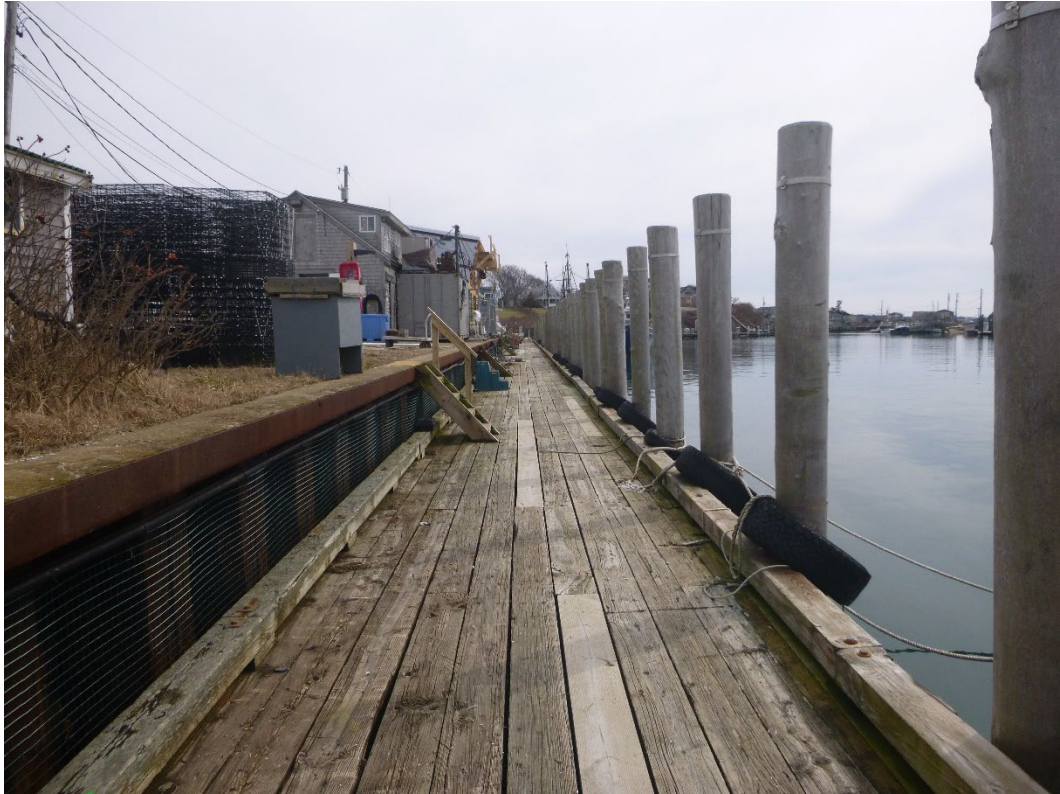
Photo 1 – Typical portion of the wharf in fair condition.
