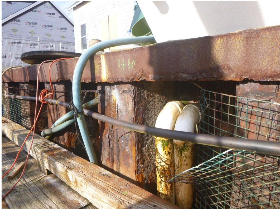
Photo 38 – Intake and outfall pipes through the sheet pile.
