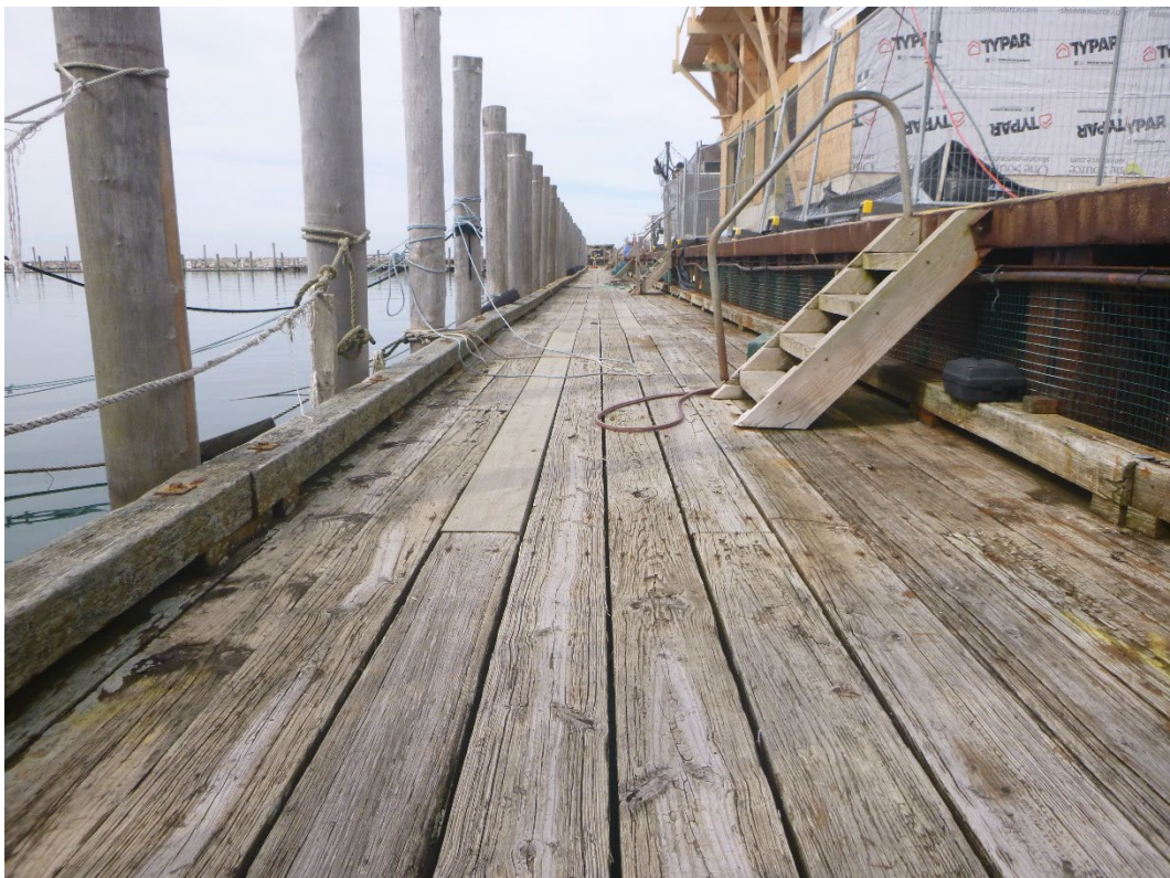
Photo 30 – Timber decking running longitudinally along the wharf.
