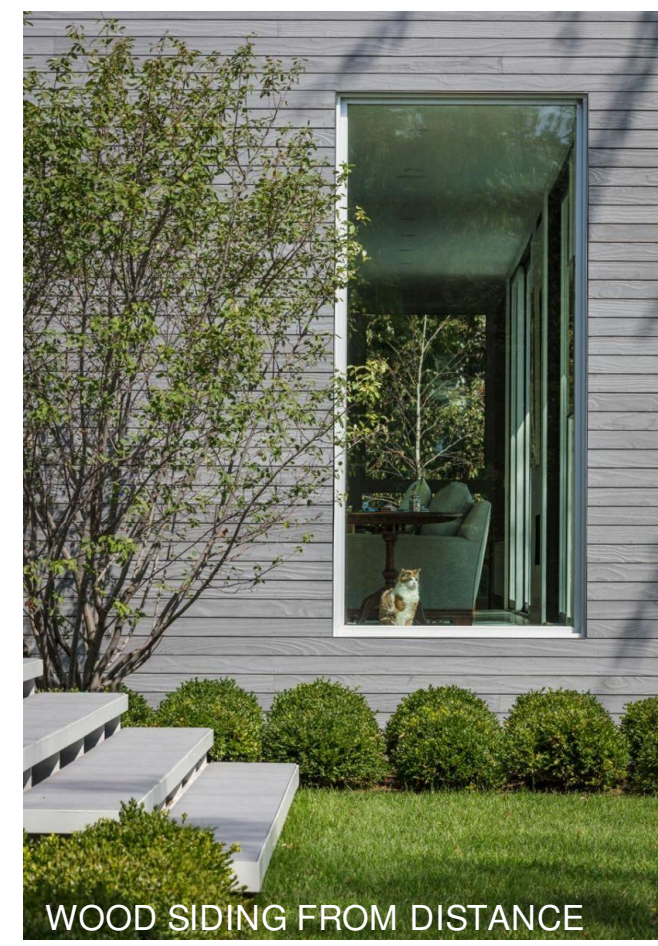
WOOD SIDING FROM DISTANCE
