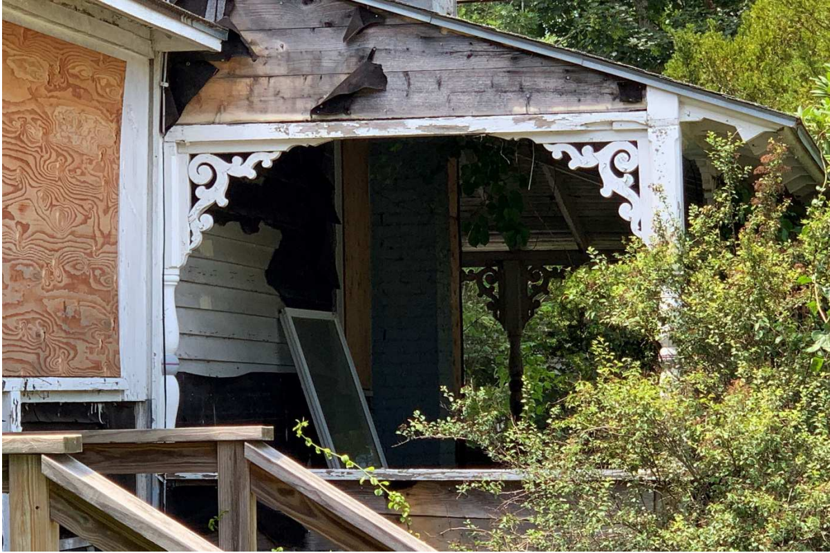
Photo 7. View of 3 Uncas Avenue left side porch from Uncas Avenue, looking NW (September 2023).
