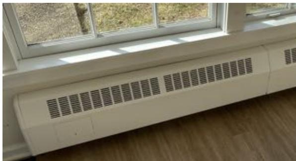
Overall, the heating system is inadequate; largely because it was never intended as the sole source of heat. The original design intent was for the finned tube radiation and the air handling units to jointly provide the heating and ventilation for the spaces. Once the air handling units were disconnected, the sole source of heat remaining was an undersized finned tube radiation system. In addition to being undersized, the layout of the radiators does not allow for complete heating coverage
